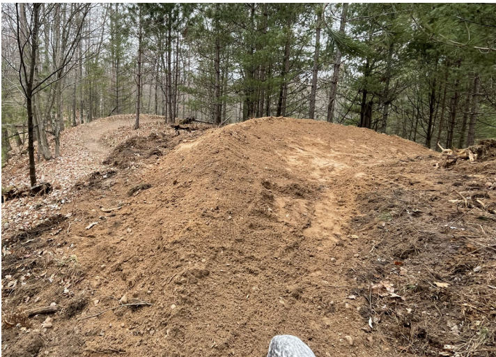
A berm under construction at the Zip Trail in Minocqua, WI.
